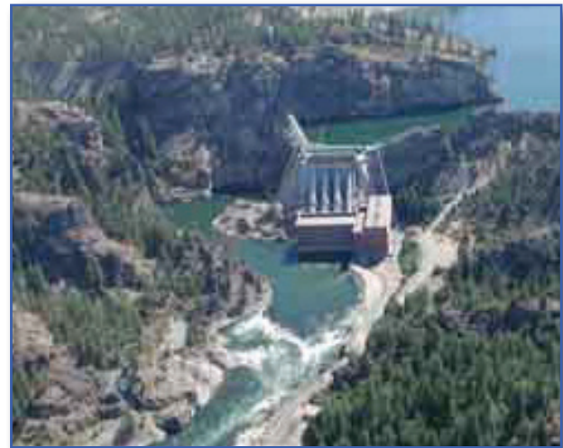
Avista's Long Lake Dam
