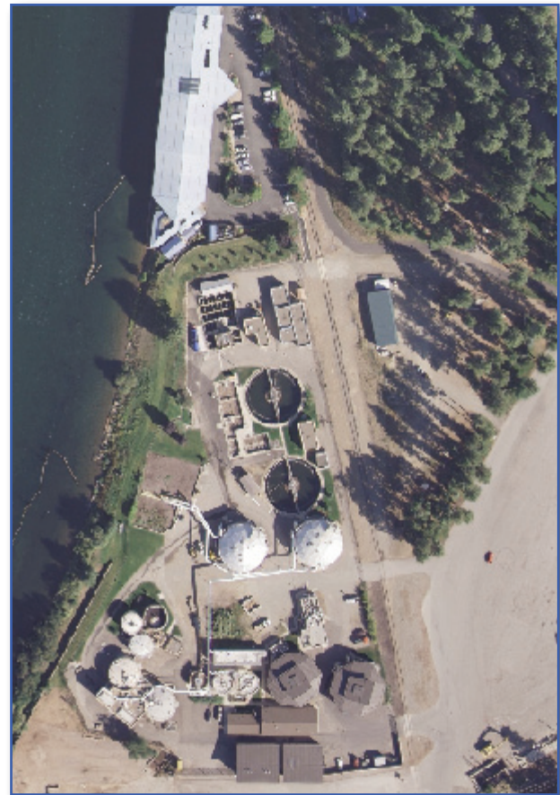
City of Coeur d'Alene Wastewater Treatment Plant
